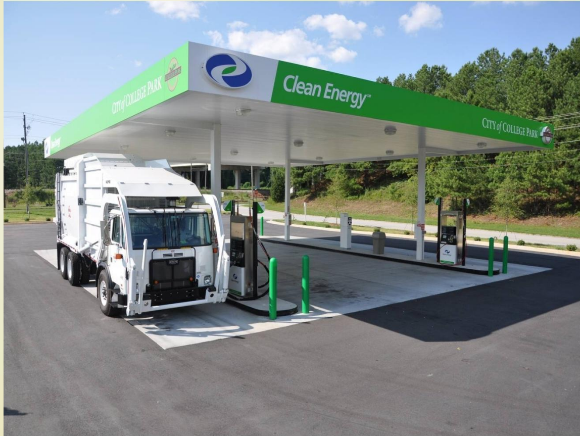
CNG facility located in Georgia
