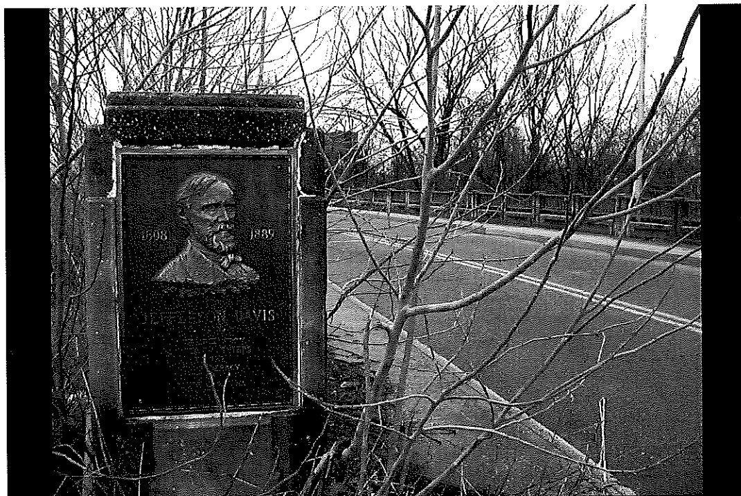
5 th Street Bridge across Savannah River?
