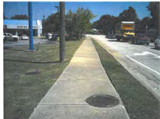
Figure 7-6. Steep Cross Slope.
