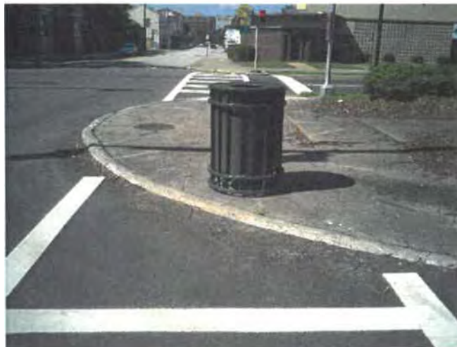
Figure 7-15. Blocked Curb Ramp.
