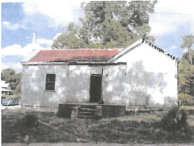
Photo 1 – 602 Weed Street in Augusta, Georgia.
