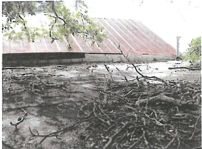
Photo 2 – Roll roofing shingles on residence.
