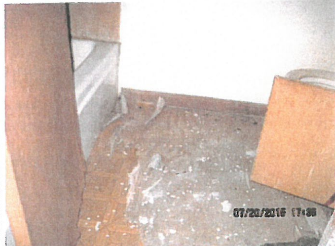
Photo 6 – wood pattern vinyl floor with no mastic.
