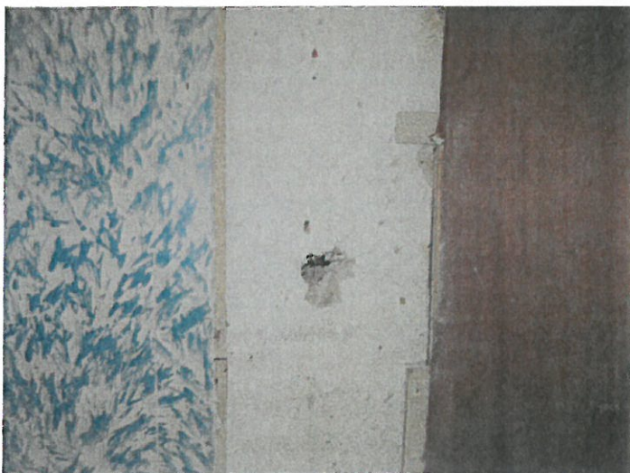
Photo 6 – Textured wall paint behind wooden wall panels.
