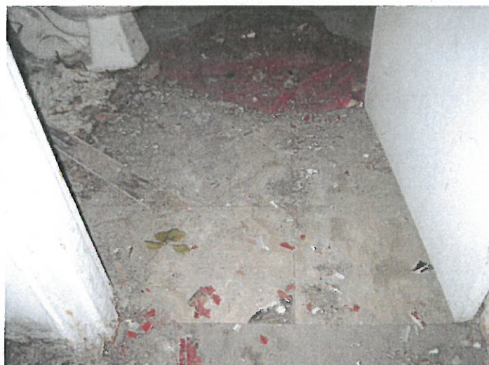
Photo 4 – 12" x 12" tan pattern vinyl floor & mastic in unit 112 bathroom.
