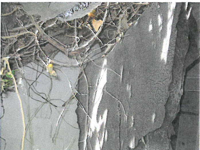
Photo 5 – Roofing material on main roof.
