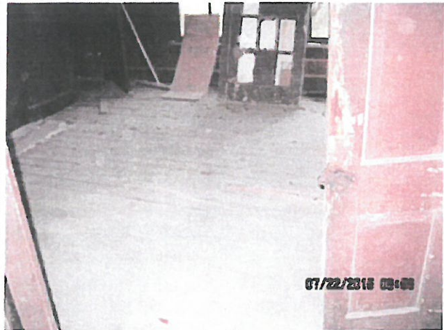
Photo 6 - Wooden floors and walls.
