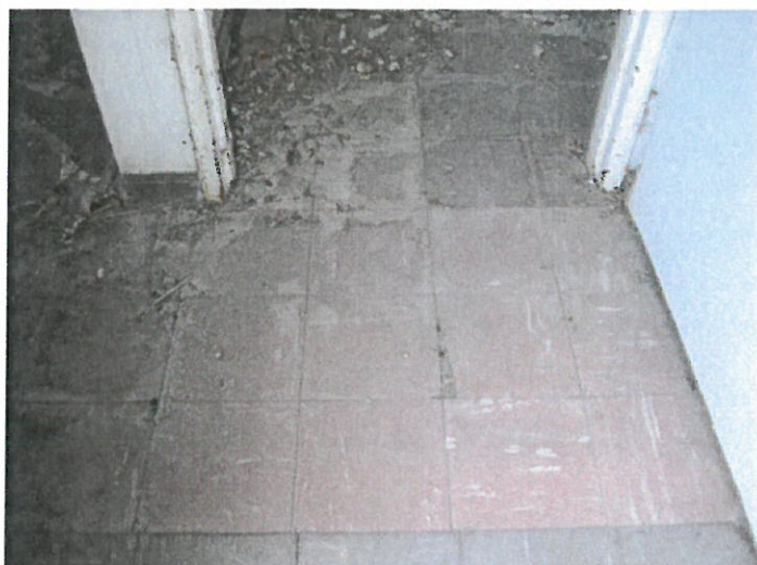
Photo 3 – Red & green 9" x 9" floor tile & mastic throughout units 112 & 114.
