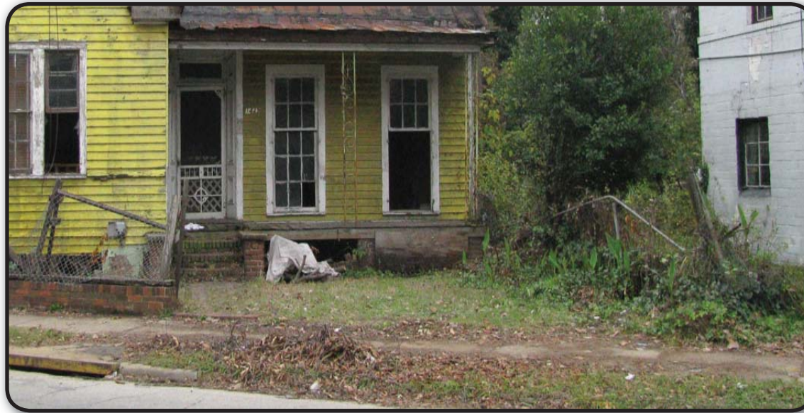
Curb and gutter with accumulated debris from insufficient drainage
